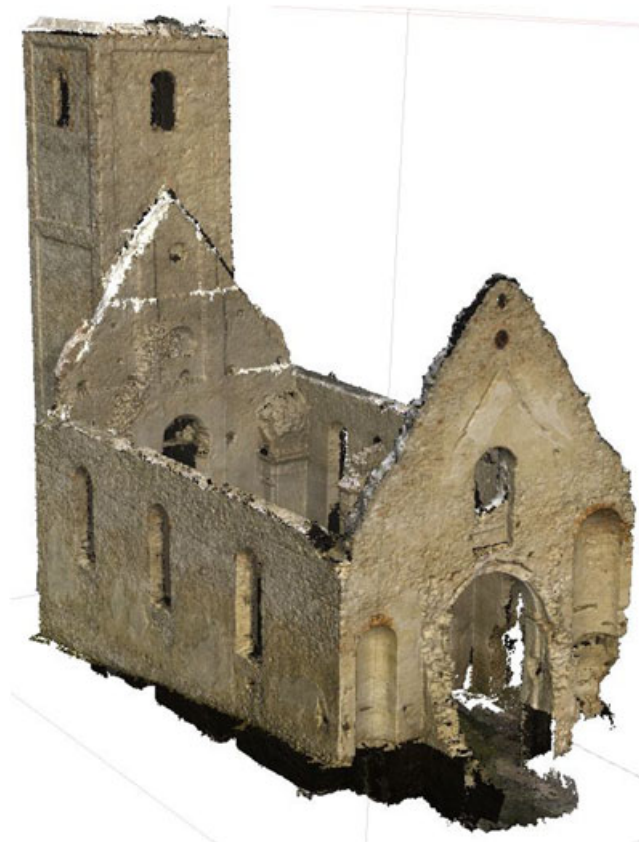
Figure 3. Three-dimensional textured model of the church, obtained by photo-based scanning. This figure is available in colour online at wileyonlinelibrary.com/journal/arp
